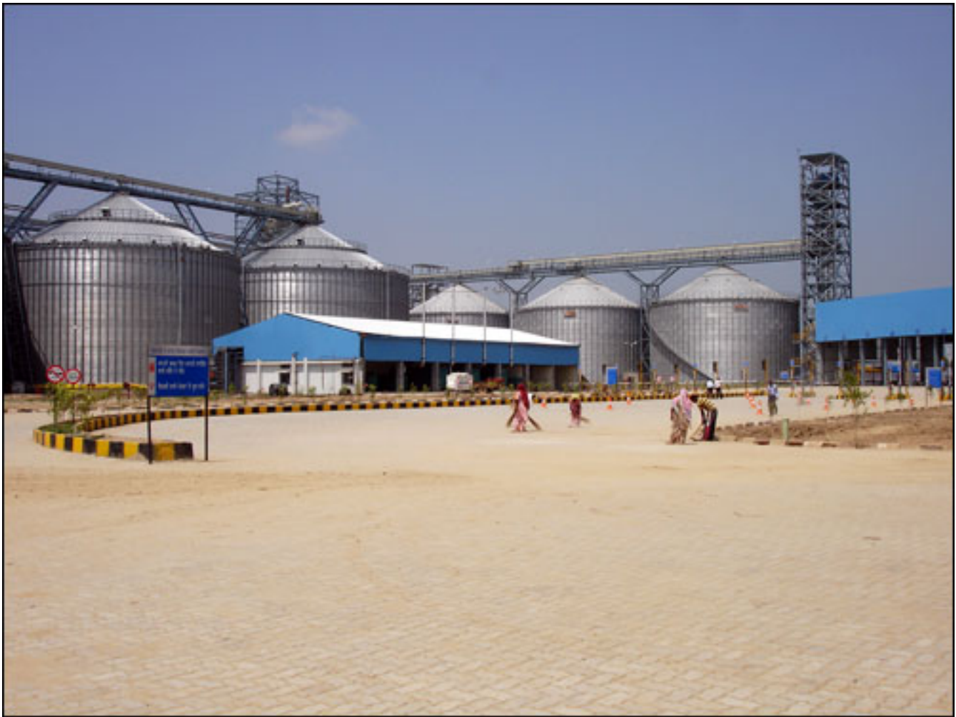
Truck lanes with silos
